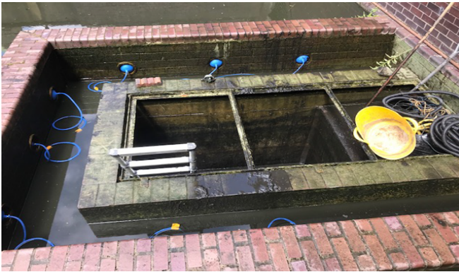
Intake pipe by The Postern – rediscovered and uncapped, after much sludge removal (almost 6ft deep)
